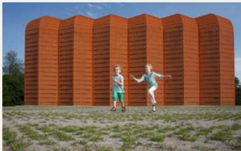
3.45 Science Park Amsterdam 150 kV station.
